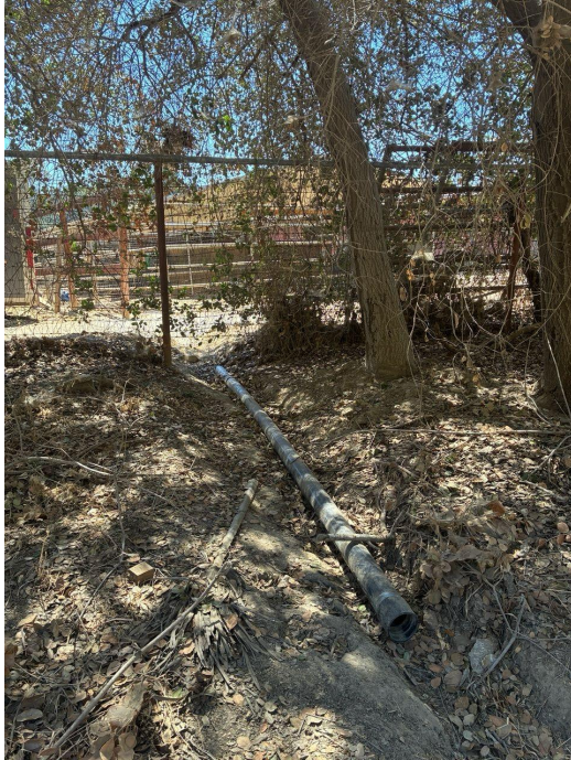
Photo 3 - San Pascual Stables piping contaminated runoff toward the Arroyo Seco.
